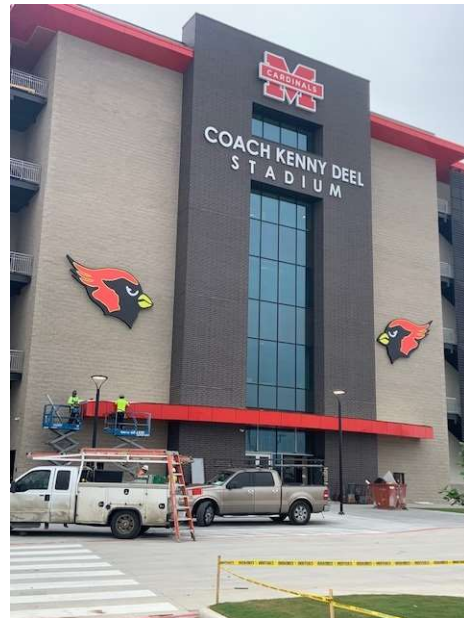
4 Separate Racks – 9 total units – Main Stadium
