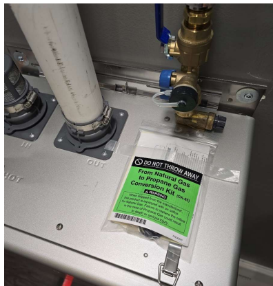
Conversion Kit taped to top of unit
