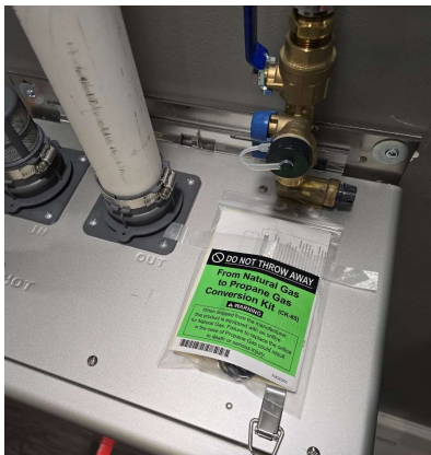
Conversion Kit taped to top of unit
